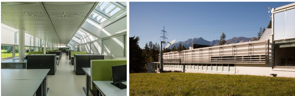
Figure 1 – Interior view of the R&D building with the glazed south façade and lowered solar shading screens (left), and exterior view of the building with the static daylight louvers (right).
